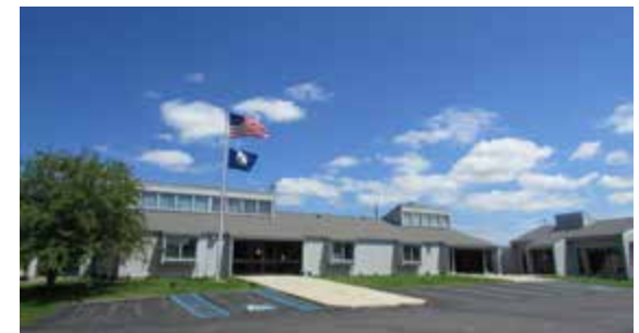
PDC Offices - Lebanon, Virginia
