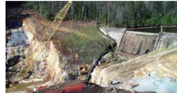
Big Cherry Dam Expansion
