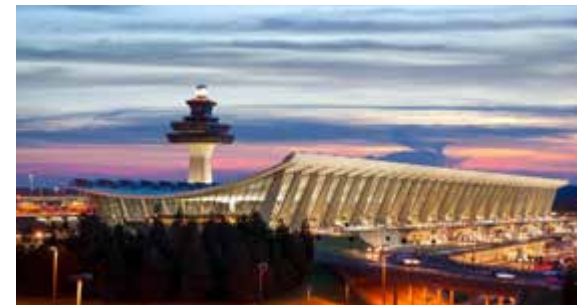
Washington Dulles International Airport in Chantilly, at dusk
